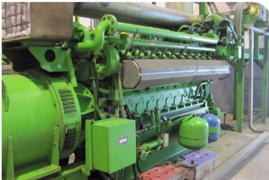
Figure 4.26: A Jenbacher 1 MW gas engine at Bantergebang
