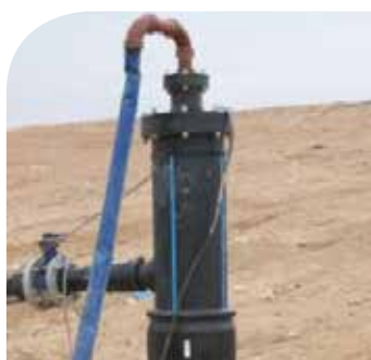
Figure 4.18: An example of a pumped well head (the blue flexible hose is for removal of leachate via a submersible pump within the gas well; gas is taken from the connection at the side and controlled using the butterfly valve)
