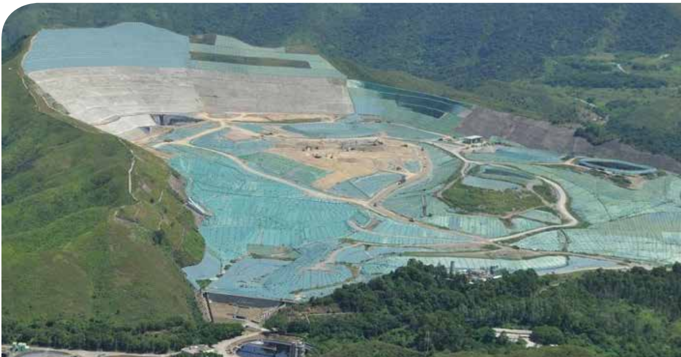
Figure 4.15: Extensive use of an interim membrane cover on a large landfill in Hong Kong
