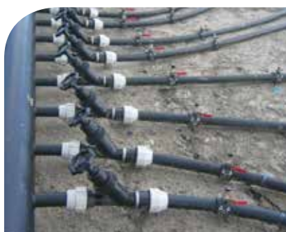
Figure 4.19: A typical manifold arrangement featuring small sample valves and larger access points for inserting flow measurement instruments
