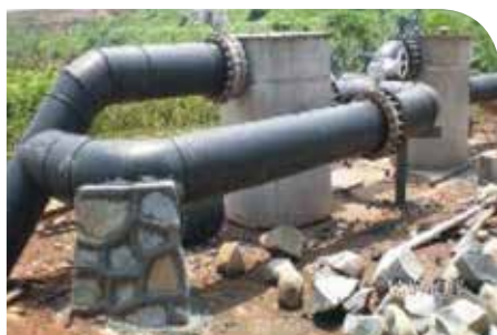
Figure 4.22: Duty and standby dewatering pots at the powerhouse, Bantergebang
