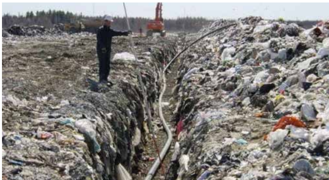
Figure 4.9: Installation of a horizontal collector in a trench, Thailand
