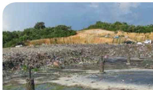
Figure 4.6: Gas wells installed prior to landfiling, Meulaboh TPA, Aceh, Indonesia
