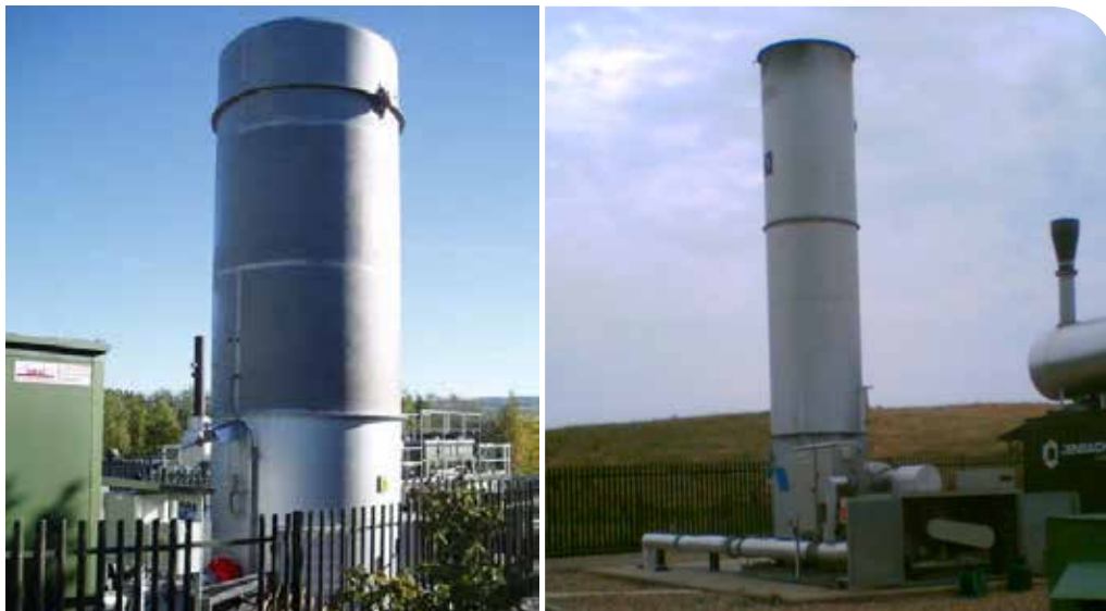
Figure 4.24: Examples of high-temperature enclosed landfill gas flares
