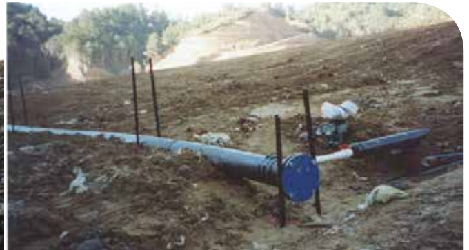
Figure 4.8: A horizontal well and collector, USA
