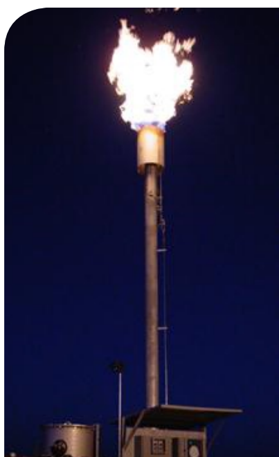
Figure 4.23: A 'candlestick', 'elevated' or 'open' LFG flare
