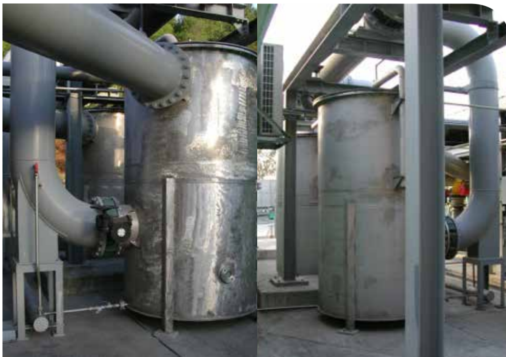
Figure 4.21: Examples of large condensate knockout pots used to deal with 10,000m 3 /hour of landfill gas in Hong Kong
