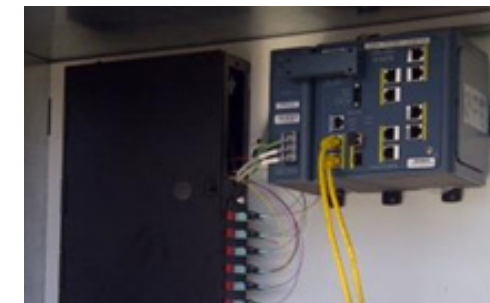
Gambar 8 Terminal Monitoring / Data monitoring di Switchgear. Sumber: Triad Engineering. Foto: Dan Jordan
